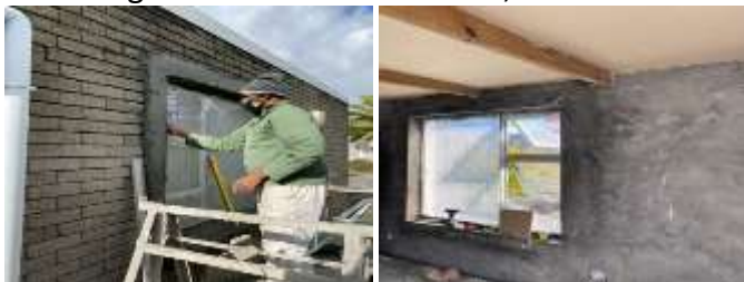
Plastering window to match estate, inside and new ceiling...
