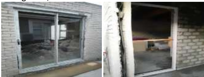
Sliding door, internal door and window...
